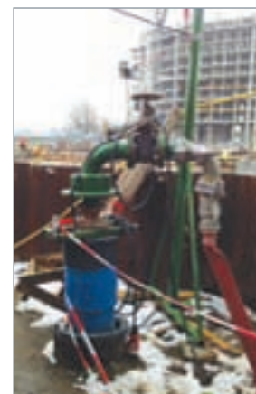
One of the completed well pairs
